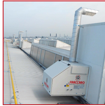
Installazione a shed Shed installation
